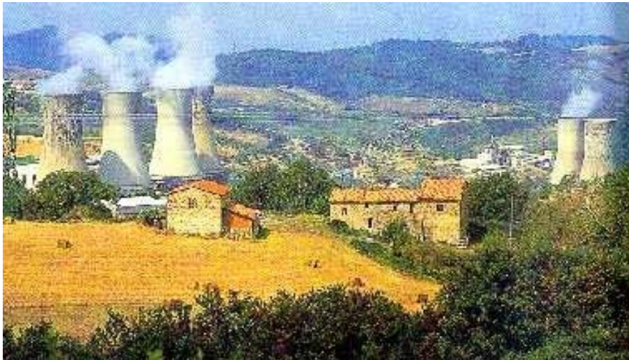
Larderello, PI Geothermal About 4.8 TWh/year
